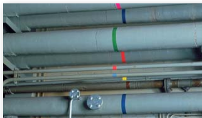
For color-coding pipes with 3M™ Vinyl Tapes, select from either nine vivid colors or transparent to let underlying color show through. Backing is colored throughout to help maintain ready visibility.
